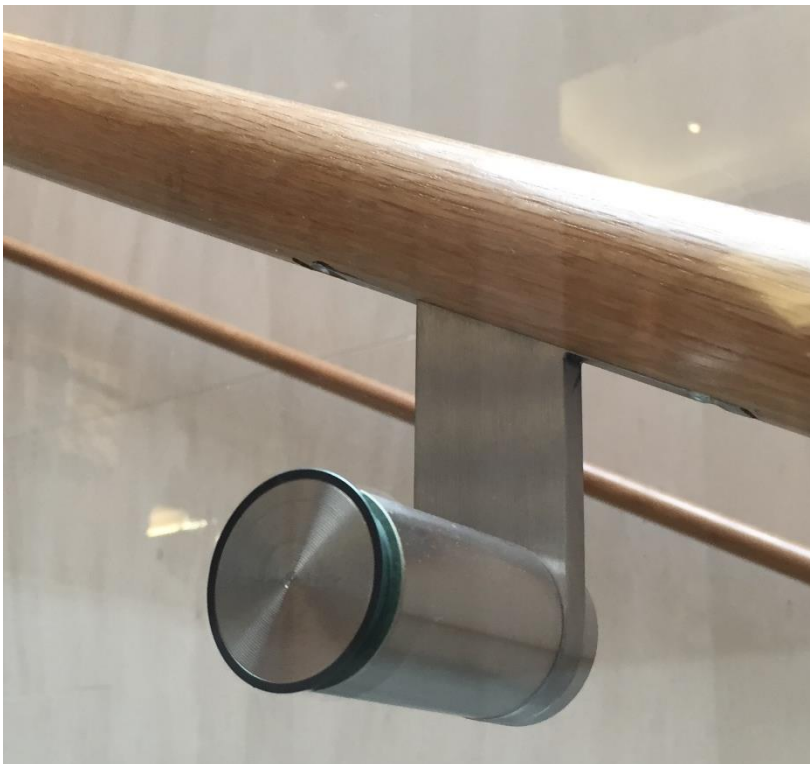
Figure 4: Embedded hardware is laminated into the glass for the handrail fittings
